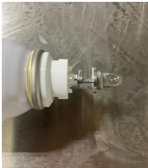
Figure 8b. Incorrectly actuated / not actuated.
